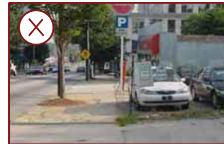
> Poor interface between pedestrian and parking, lacking a landscape buffer between parking spaces and sidewalk.
