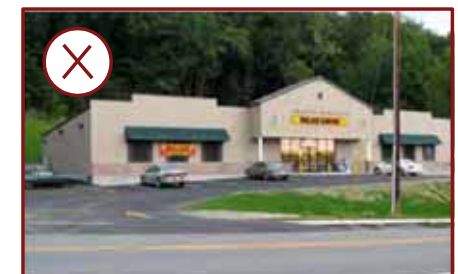
> Example of a development that does not provide adequate sidewalks and/or appropriate connections to neighboring developments
