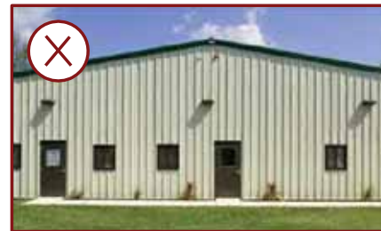
> Example of a pre-engineered metal building that is not permitted in the Gateway Corridor Overlay District.
