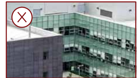
> Transparent materials such as glass should be balanced with solid, durable materials such as stone, steel, high-grade wood, and masonry.
