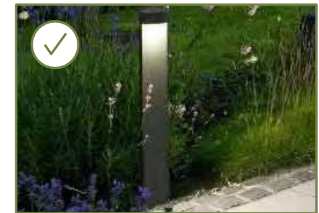
>Example of an appropriate pedestrian path light (specs shown on following page)
