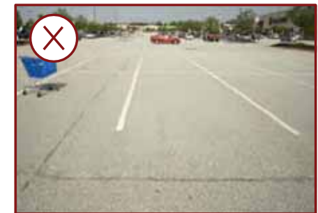
> Large expanses of non-porous asphalt parking without vegetation
